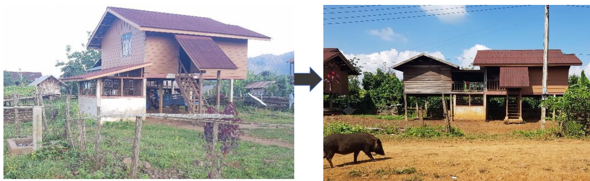
Figure 22 The HLG project-built (left) and villager-modified kitchens (right) in Ban Houay Lamphan
