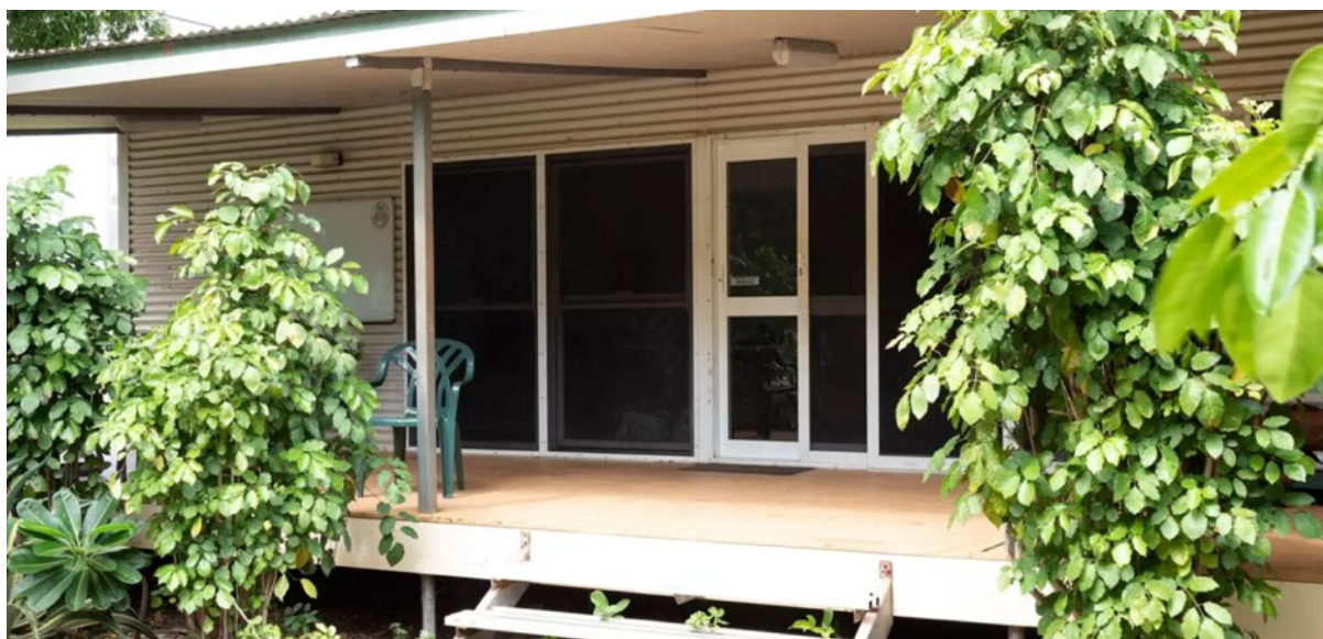
Figure 9: Visiting Officers Quarters at Bäniyala, constructed 2007
