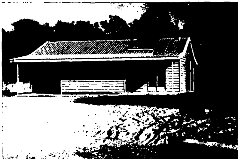
A Miriwoong design and construction
