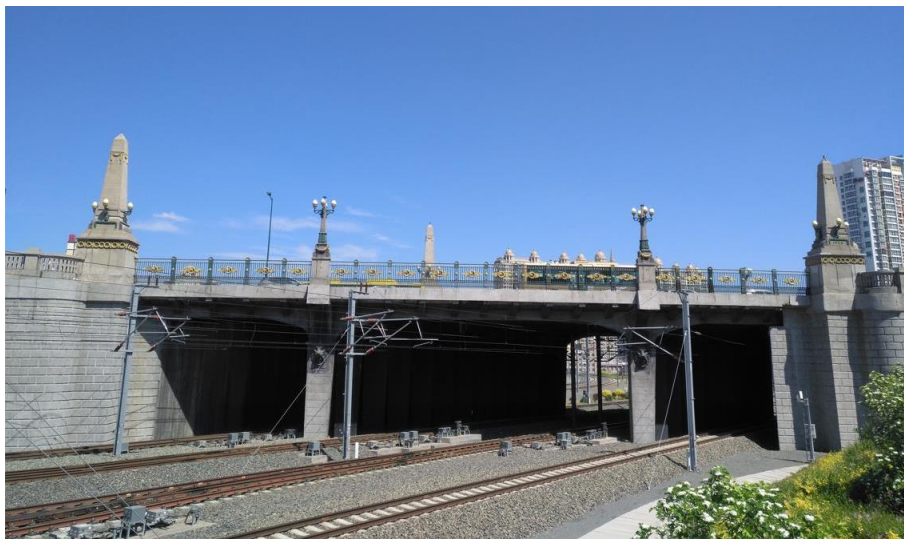
Figure 4.3 The transformed Jihong Bridge
