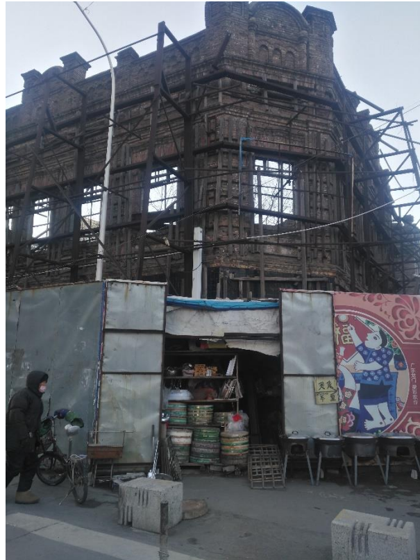
Figure 4.7 A ‘nail household’ in a mostly demolished Chinese Baroque building
