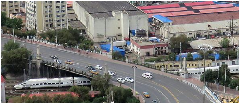
Figure 4.2 A high-speed train passing under the original Jihong Bridge
