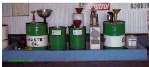
Figure 2: banded liquid waste storage with full waste separation for recycling.
