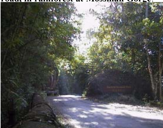
Figure 1: Town water pipe beside the road, in rainforest at Mossman Gorge.
