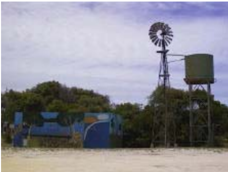
Figure 2: Beachside toilet block managed by Albany City Council
