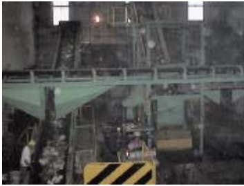
Figure 1. Waste sorting in the Atlas Plant, Stirling City.
