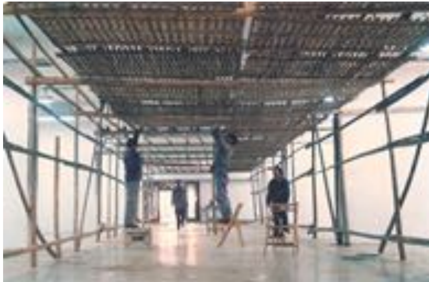
Figure 47. The construction of the passageway for The Last Supper performance in December 1988.
