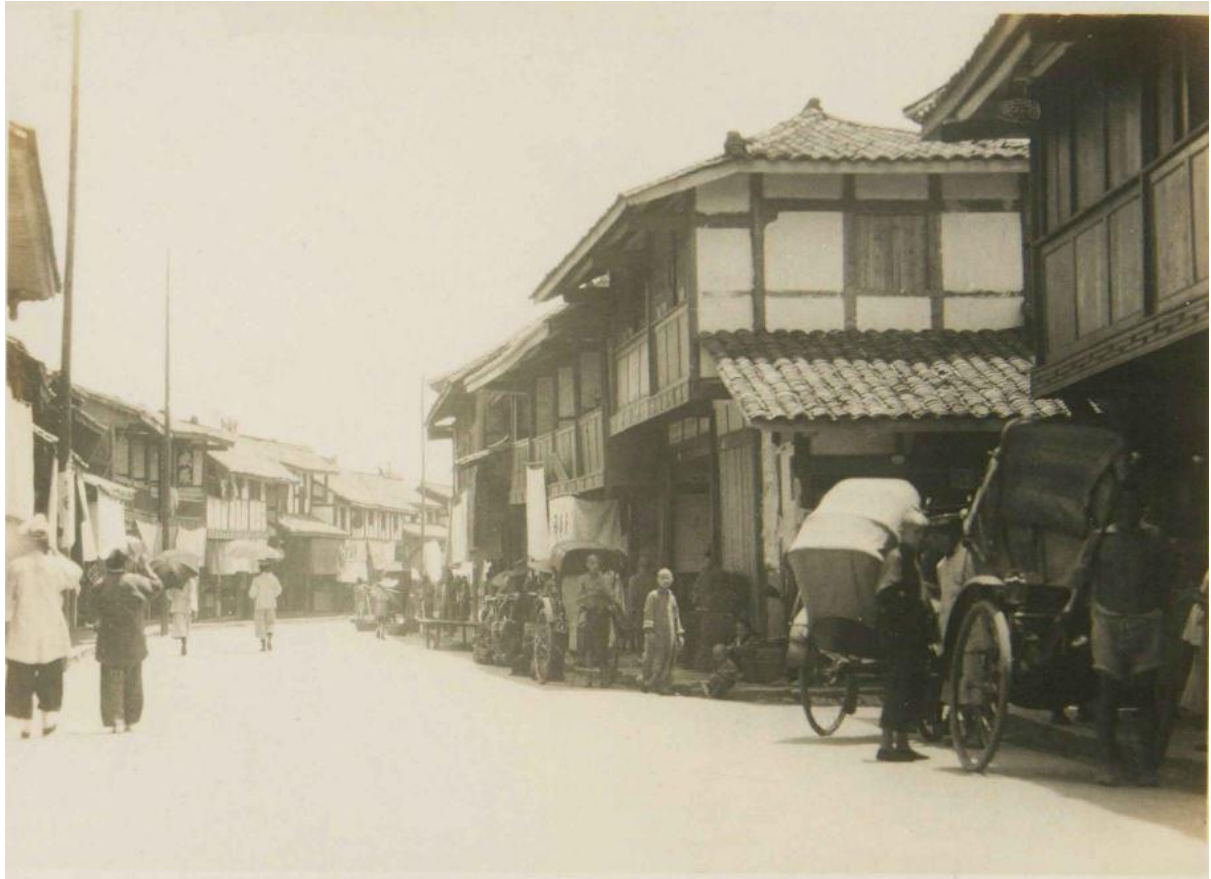
Figure 3.6 The streetscape in the 1920s. This photo was captured by Daoqi Yizhi. Source: Kokuryūkai Shuppanbu (1928, No. 566).
