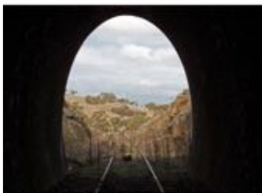
Francis, K. (2012). Scotsdale Tunnel view: digital photo.
