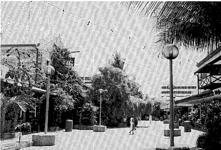
Plates 7 and 8: Smith Street Mall - under construction (above) and completed (below).
