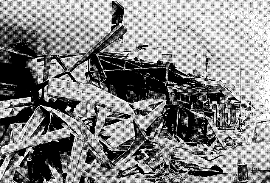
Plates 5 and 6: Smith Street Darwin - before Cyclone Tracy (above) and after Cyclone Tracy (below).
