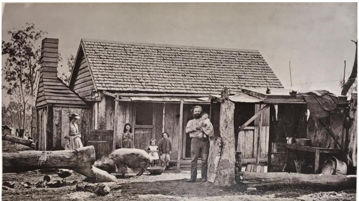
Figure 6.2 Free selector’s slab hut Plate 12 Richard Daintree Queensland, Australia. Its Territory, Climate and Products
