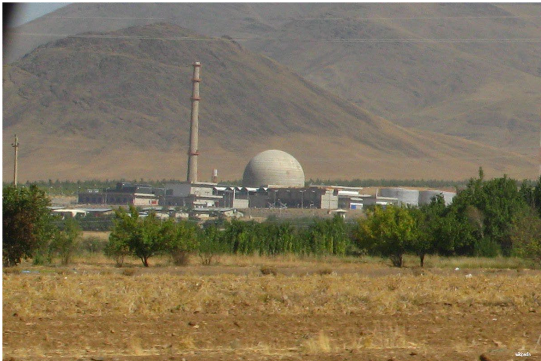
The dome of the reactor in the foothills of the mountains surrounding Arak
