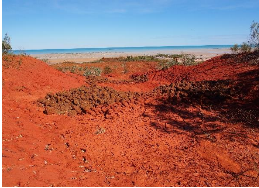
Figure 9.6: Erosion mitigation measures at Crab Creek. Rocks placed to prevent vehicle access and slow erosion in a high erosion area (left). Sumps installed adjacent to the east-west road to prevent run-off and water pooling on the road (right).
