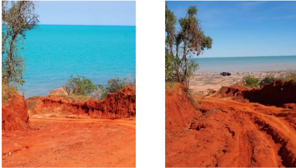
Figure 9.5: Erosion of the Sabu Rock access track. The image on the left was taken in May 2015, the image on the right was taken in June 2017. Considerable erosion took place over that time.
