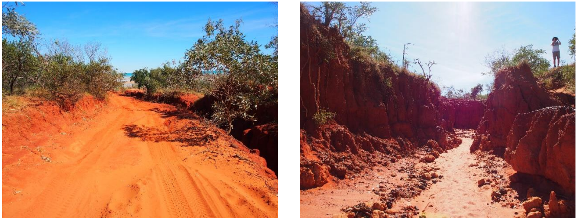
Figure 9.4: Deep gully erosion at Crab Creek. The image on the left shows the top of deep gully erosion adjacent to an area used by vehicles to access the beach. The photo on the right shows the same gully, but taken from the beach.
