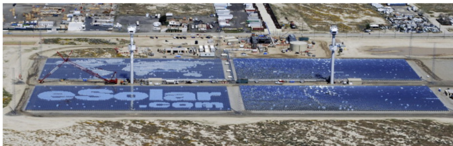
Fig. 1.4: Sierra Suntower Demonstration facility, Lancaster, CA, USA in April 2009. Source extracted from [23]
