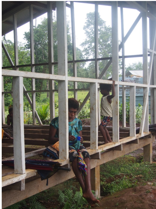
Image 2: Classroom construction, Pomio, East New Britain.
