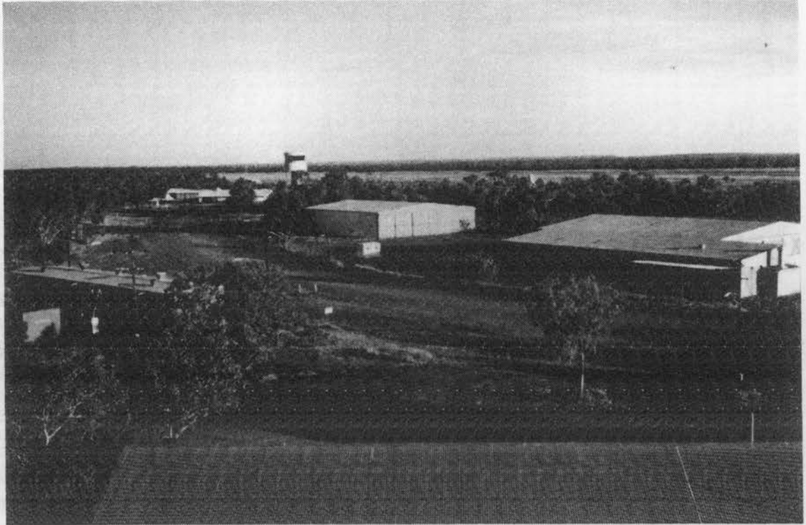
Plate 3.1 A view of the facilities constructed by 5 ACS also showing the completed control tower for the new development.
