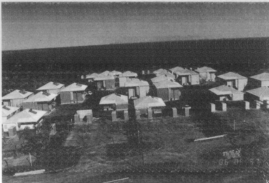
Plate 3.4 A view of the on-base accommodation for the living-in single personnel at Tindal RAAF Base
