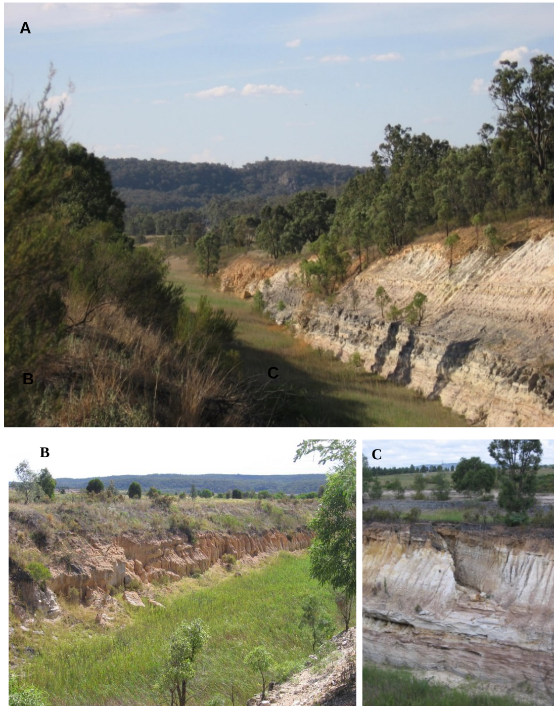
Figure G1 - Goulburn River Diversion (2004) A) main channel looking north-west B) undercut bank erosion C) erosion of highly dispersive clays
