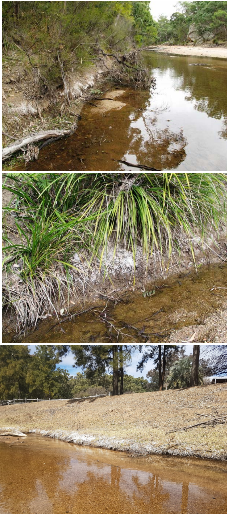
Figure G2 Goulburn River @ Gleniston Site (21010017) – encrustations of evaporated salts deposited by capillary action during a period of low rainfall (Photo: 4 August 2013 & 12 September 2017)
