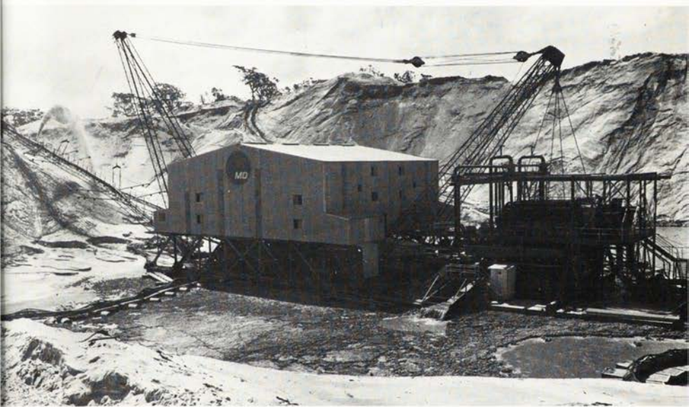
Below: Mineral Deposits' 1500 tonnes per hour operation. By courtesy of Mineral Deposits.
