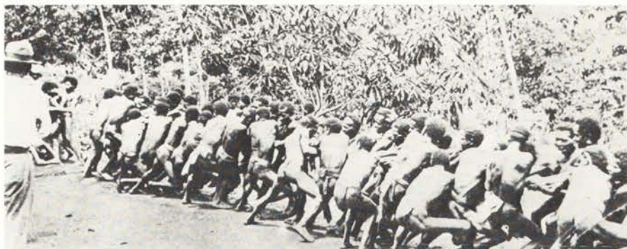
XII Men bringing a wharf pile into position at Ogamobu plantation, Kikori River, 1920. From A Pictorial History of New Guinea by Noel Gash and June Whittaker, Jacaranda Press
