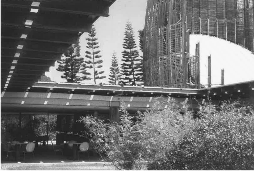
Figure 3 Looking from Kanak path into the Péruï House and cafeteria area, the Centre Culturel Tjibaou, Noumea. Photograph by Kylie Message. (Courtesy of the ADCK-Centre Culturel Tjibaou/Renzo Piano Building Workshop, Architectes.)
