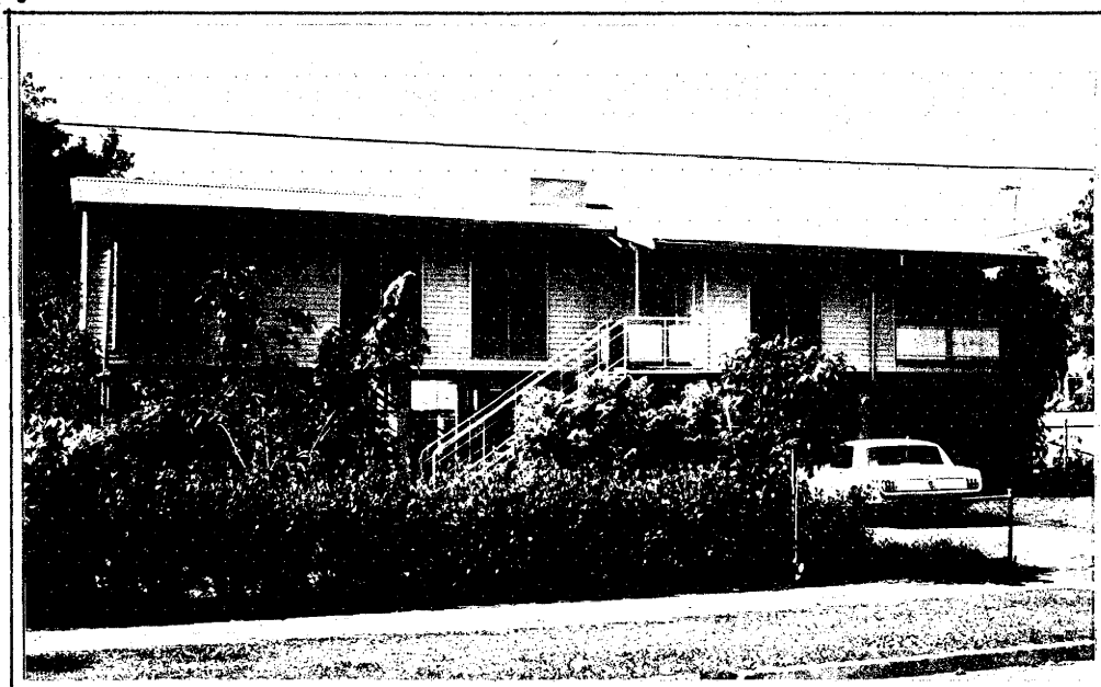
FIGURE 23 Damaged "M" type house.
