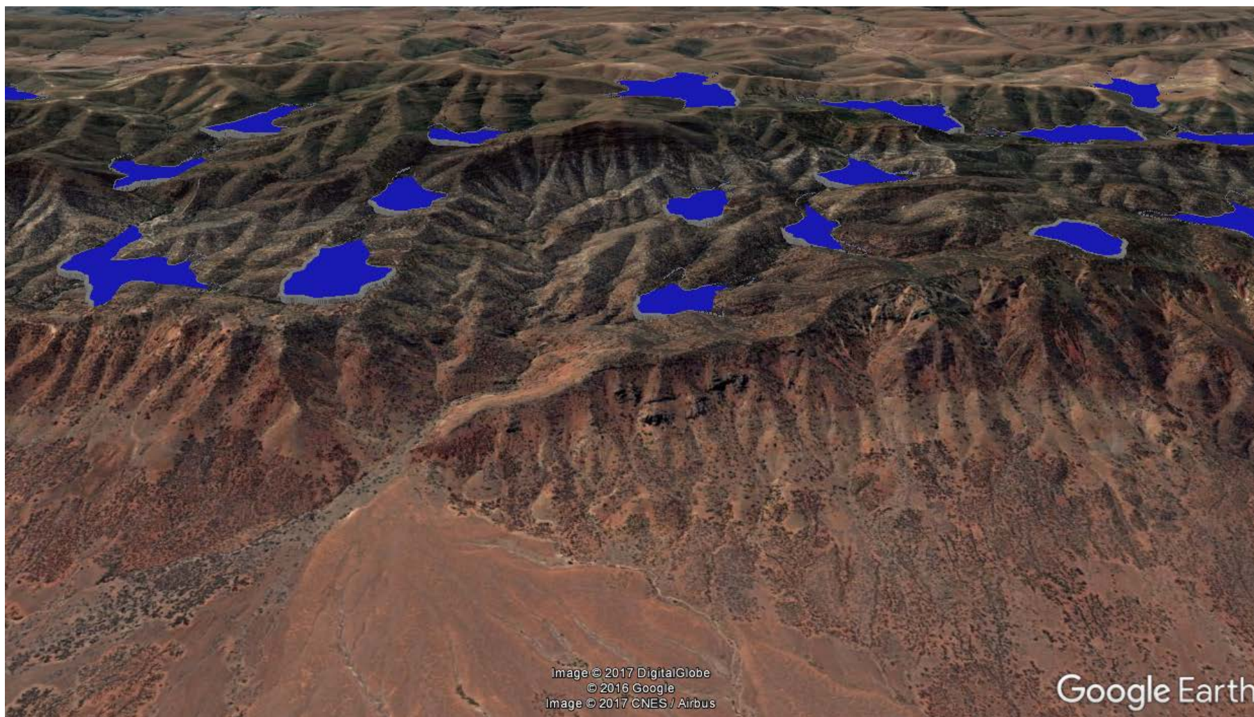
Figure 2: Potential PHES upper reservoir sites in Region A, east of Port Augusta. The lower reservoirs would be at the western foot of the hills (bottom of the image).
