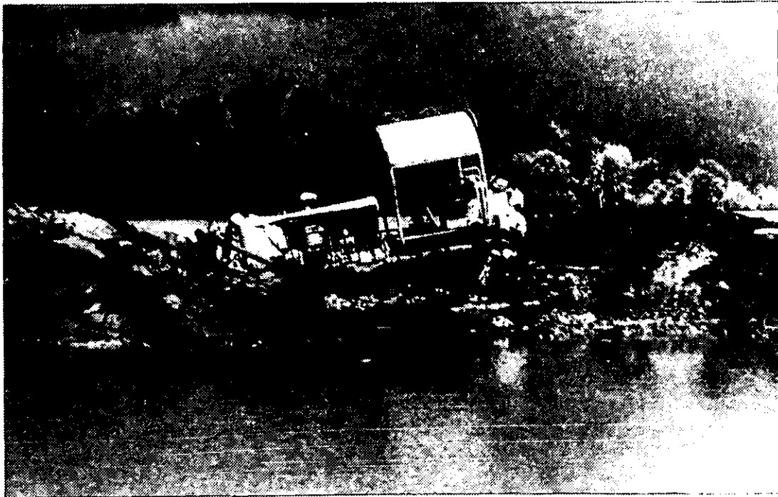
2. This RAAF bulldozer has become bogged while building earthworks where water was to be pumped from the river. Delays of this sort frustrated attempts to keep to work schedules. The cloud cover poses another threat.
