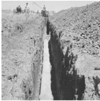
Pipeline construction, Robinvale irrigation settlement, 1957, State Rivers and Water Supply Commission. Courtesy: State Library of Victoria
