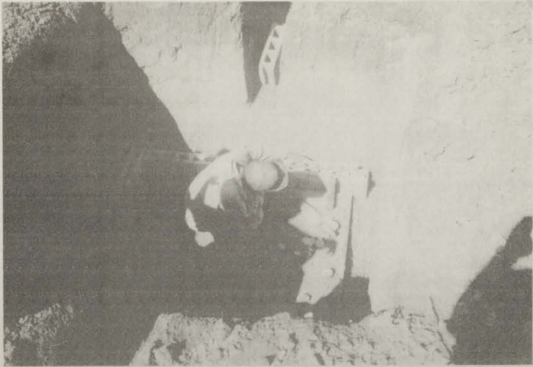
Putting of iron rods into the holes of the blocks
