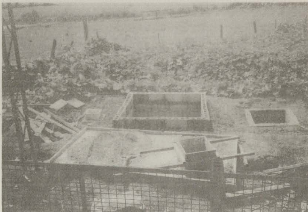
Cementing of the floor of fermentation tank
