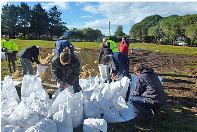
Figure 4. AHSPP team filling more sand-bags for stabilising the site (Photo: J. Rodrigues).
