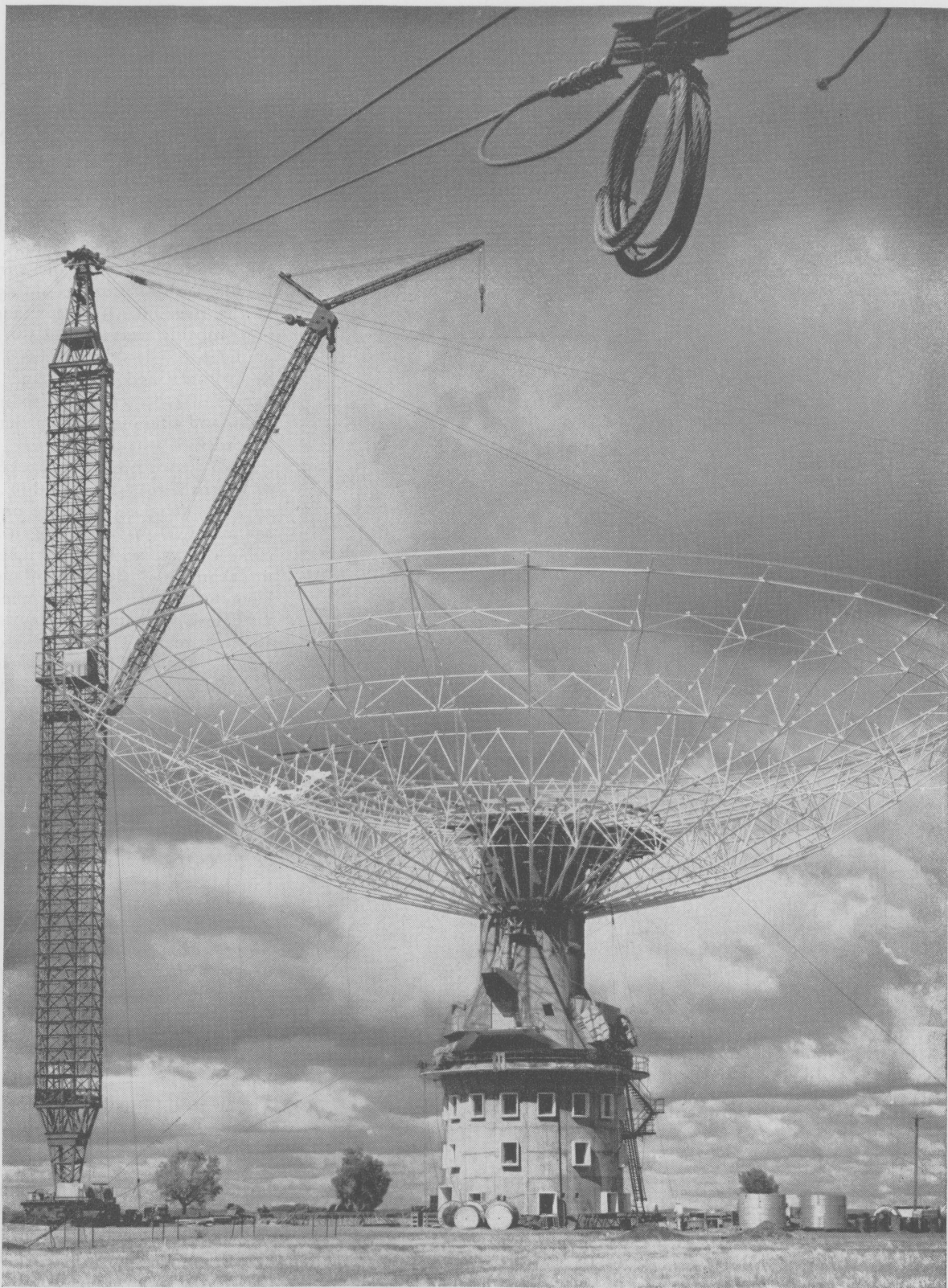
The world's second largest steerable radio telescope, during construction of its 210-foot paraboloidal radiation collector. It is being erected at latitude 33^{\circ} south, near Parkes, New South Wales, Australia, by the Commonwealth Scientific and Industrial Research Organization, for studies of the Milky Way and other galaxies. Photo from Radiophysics Division, C.S.I.R.O.
