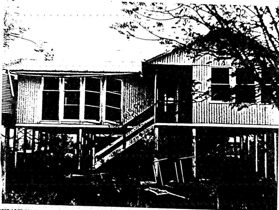
DEGRADED DWELLING - YUENDUMU N.T.
