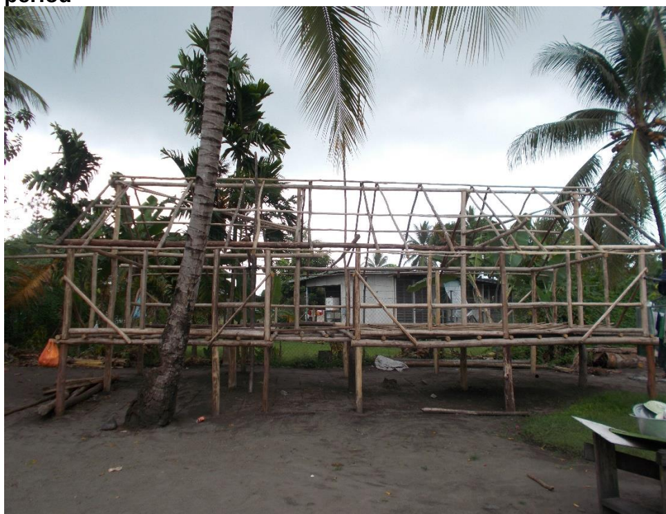
Photograph 7-9. A new haus win under construction at Lucky Base for election period
