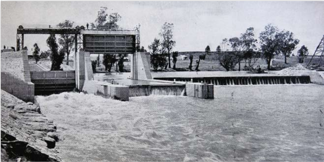
Plate 13.1 Berembred Diversion Weir and Lock (in Brady 1911: opposite page 178).
