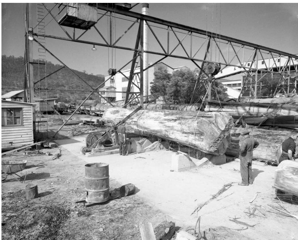
Figure 5 A tree is processed at the Australian Newsprint Mills factory at Boyer, Tasmania, c. 1952. The trees were fed to pulping machines that converted them into the light, cheap paper relied upon by newspaper publishers. AB713/1/992, Tasmanian Archives, Hobart.
