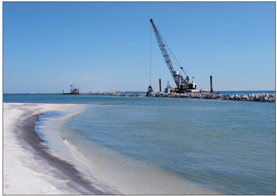
Figure 3. Crews blockade the inlet with riprap at Katrina Cut on Dauphin Island, Alabama. This view is from the uninhabited west end of the island, looking across the inlet toward the heavily developed east end.
