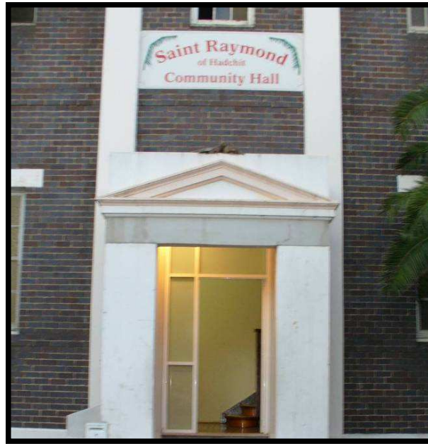
Figure 19: The St. Raymond of Hadchit Community Hall in Granville. Source: Nelia Hyndman-Rizik, 2006.
