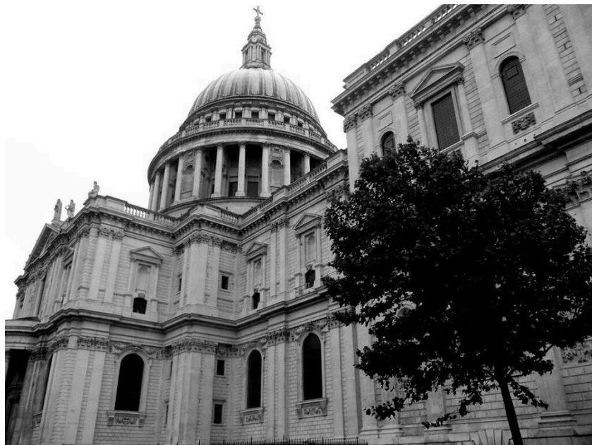
Figure 4: The famous dome of St. Paul's Cathedral, London. The present building was constructed in the English Baroque style by Sir. Christopher Wren in the 17 th century.
