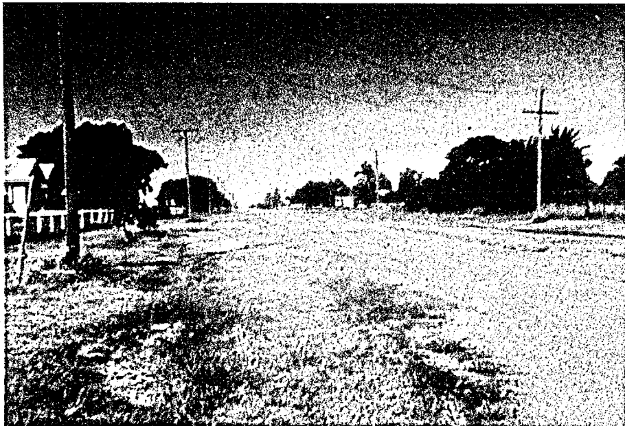
Gidyea Street-a section of unsealed town street with wide verges and no kerbing.
