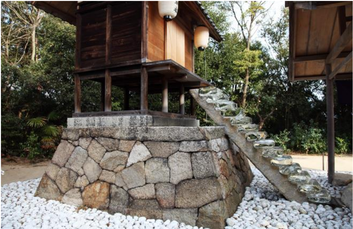
Figure 100: Picture of the glass stair leading to the Honden (Shrine), the Haiden (Hall of worship) is on the right hand side (photograph by author)
