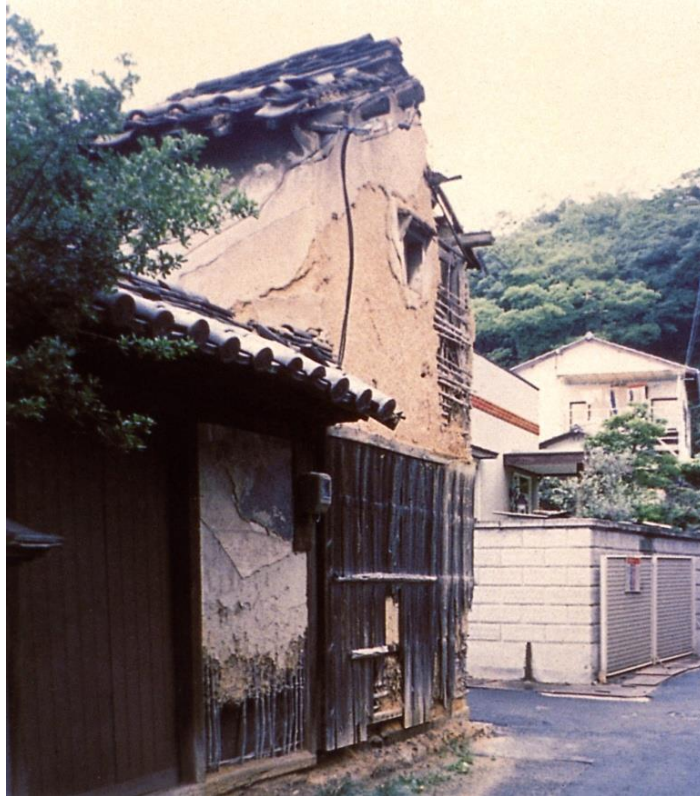
Figure 61: Kadoya Art house site prior to renovation
