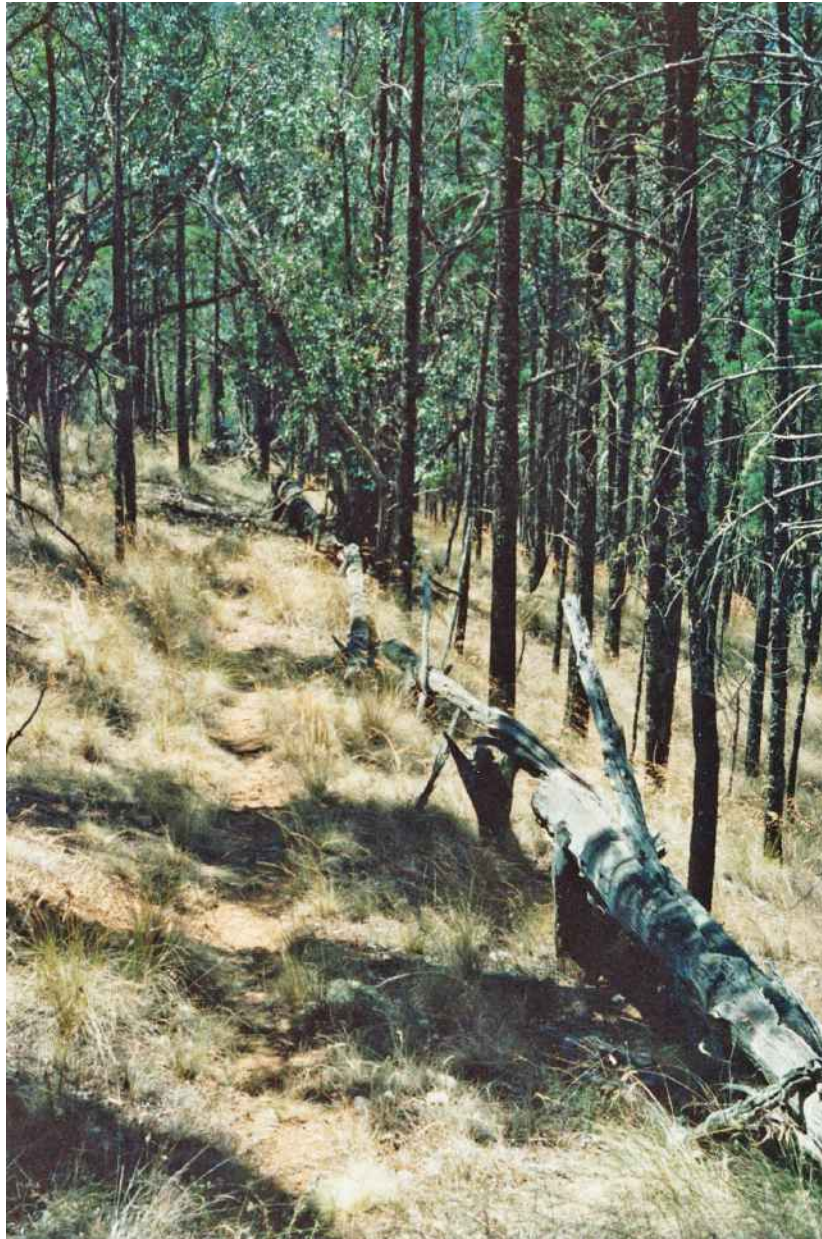
Plate 3.1 Remnants of an old timber fence around Mount Trooper built before c1900 which was constructed of white box supports and white cypress pine rails. No other materials were used in construction. The existence of the fence is evidence that fire has not burnt these slopes this century.
