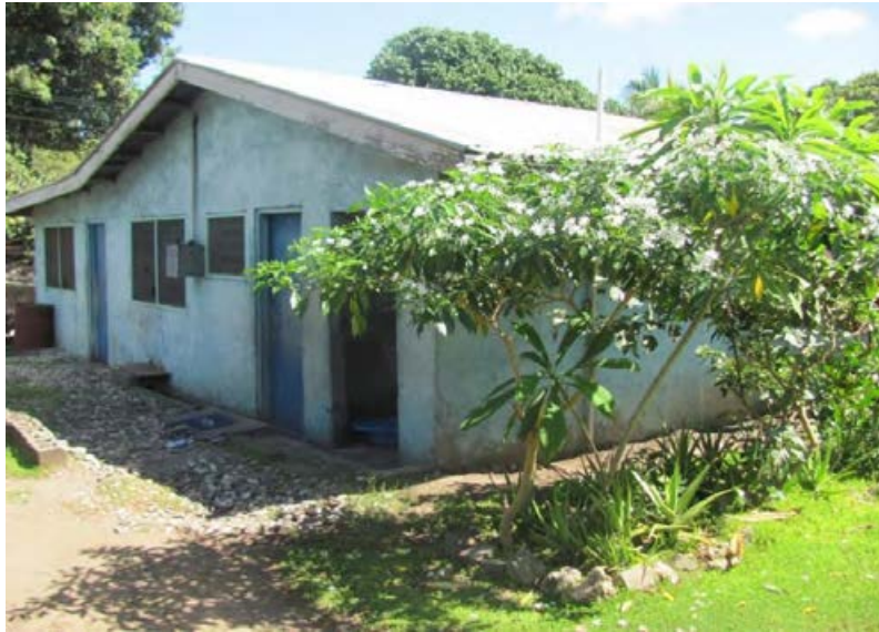
Figure 8.3: Mamaloni's single quarters at Kukum, with external toilet, shower, and kitchen. Source: author.
