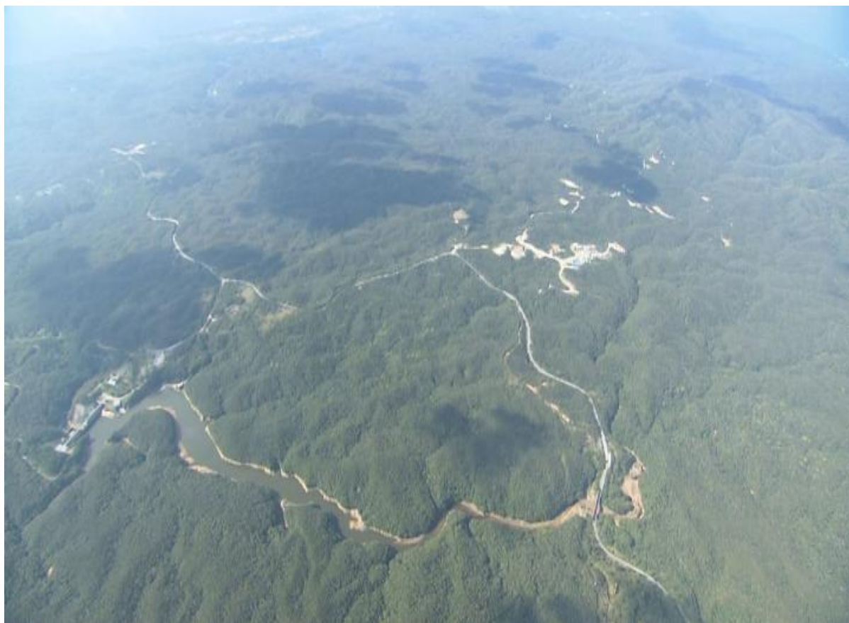
Image 5-2: An aerial view of construction sites. On the bottom of the left is Arakawa Dam. The photo was retrieved from the website of the Okinawa Prefectural Government. ( http://www.pref.okinawa.jp/site/chijiko/kichitai/1172.html , accessed, July 16, 2015)
