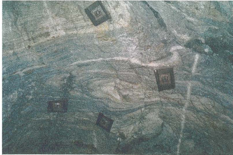
Figure 4.2 – Mylonite zone in the marble. Photo taken of backs on 10400mRL level. Rock bolt plates are approx. 40cm.
