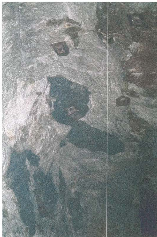
Figure 4.3 – Photo of blocks within the mylonite zone. Dark blocks are volcaniclastic and top right corner shows block of skarn altered material. Photo taken of backs in 10400mRL level. Rock bolt plates are approx. 10cm
