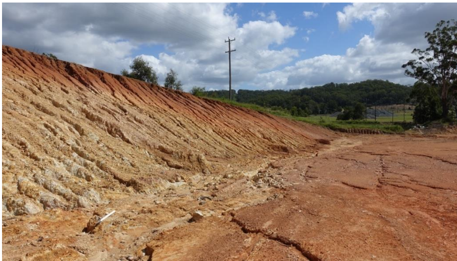
Plate 13. Borrow area at Cobaki Lakes, a development site the subject of litigation in Secretary, Department of Planning and Environment v Leda Manorstead Pty Ltd (No 2) [2018] NSWLEC 195 in which the data sufficiency relating to erosion and sediment was contested. An expert witness retained by the prosecution collected no data and was obliged to rely on data collected on behalf of the defence (Photograph by author, 2017).
