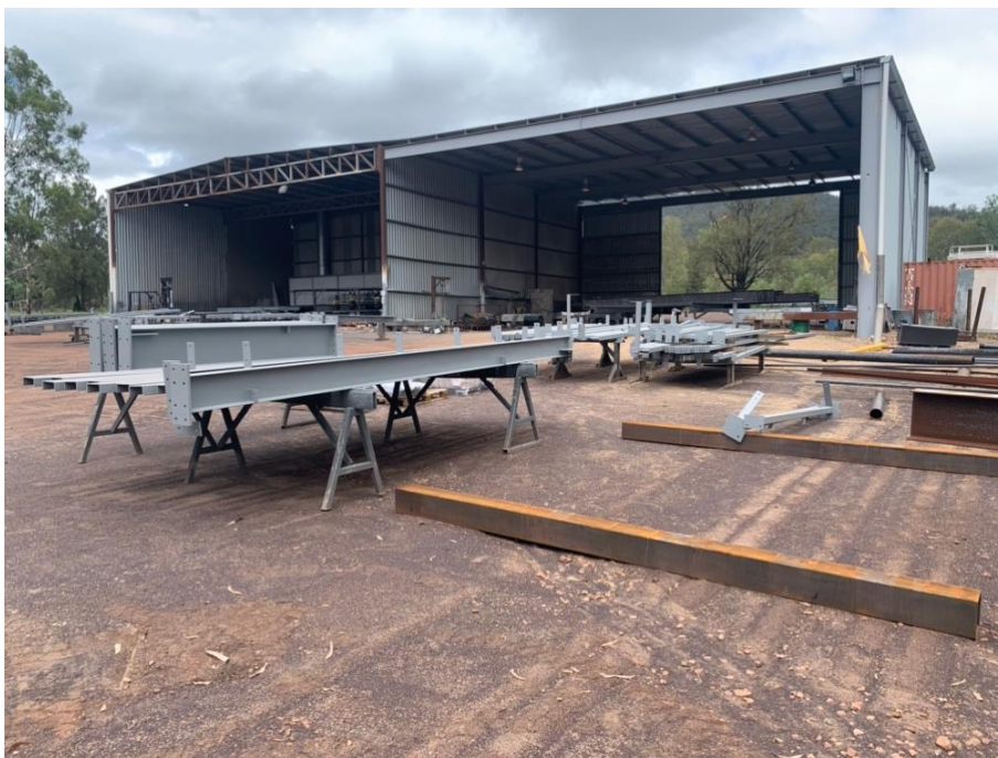
Plate 12. Steel fabrication workshop in Widgee, Queensland, the subject of a dispute with downstream neighbours and the local authority, Gympie Regional Council. The dispute centred on contamination of lands downstream of the facility. The issue was resolved, in part, by testing upstream of the workshop in a catchment that had been formerly mined. (Photograph by author, 2020).
