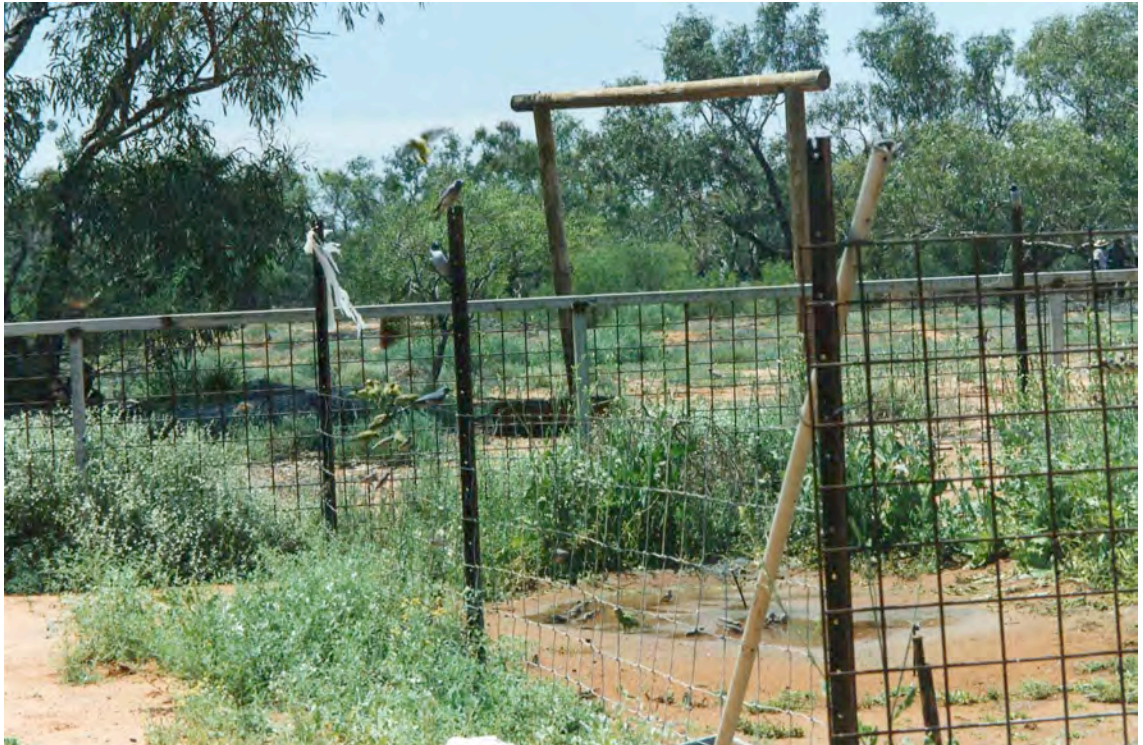
Fig 1.8: Preparation for vegetable garden and lawn, irrigated with bore water at Oasis Bore. 'Two houses, grape, fig, passion fruit and gum saplings planted. Lawn under shade cloth at front of the house. Fence not finished, generator not here yet.' (Macfarlane field notebook 9/7/96).
