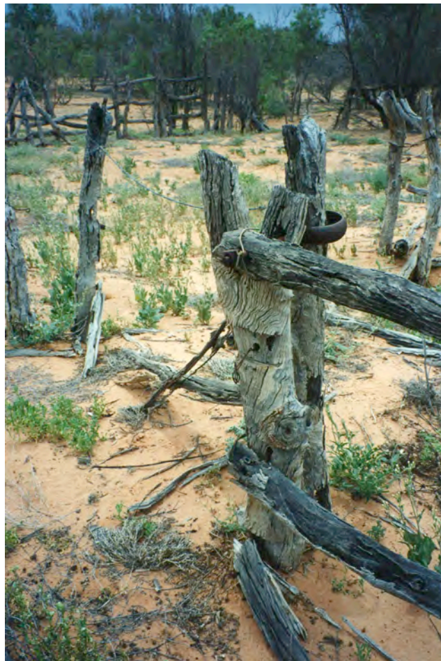
Fig 1.4: Smiths Yards (construction detail), September 1997
