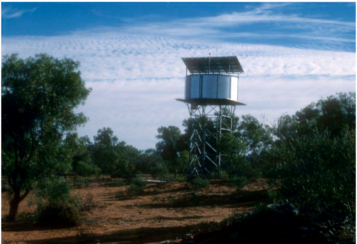
Fig 4.15: New tank with solar panels at Anniversary Bore, October 1997
