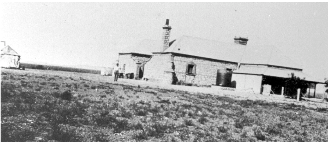
Fig 2.28: Back of the telegraph station, a post office in c1920, SLSA B45180
