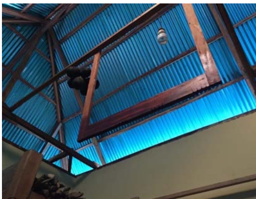
Plate 20 Above the hearth, wooden walls give way to concrete and a corrugated metal roof.
