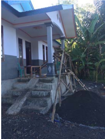
Plate 71 The unfinished house.
