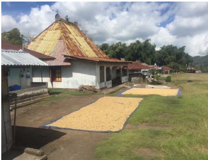
Plate 22 A large concrete building containing a sa'o , Bogala.
