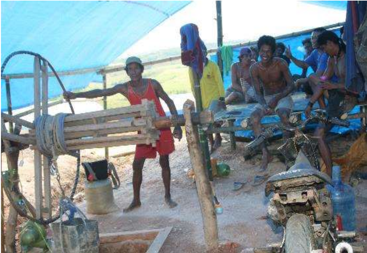
Figure 3.12 A vertical rat hole with winches, blower, ropes and cans used to signal that the materials or people are ready to be lifted up
