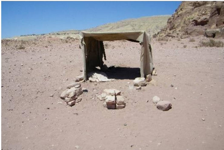
Basma Faqyra' shop before she renovated it and replaced the hessian with tent cloth
