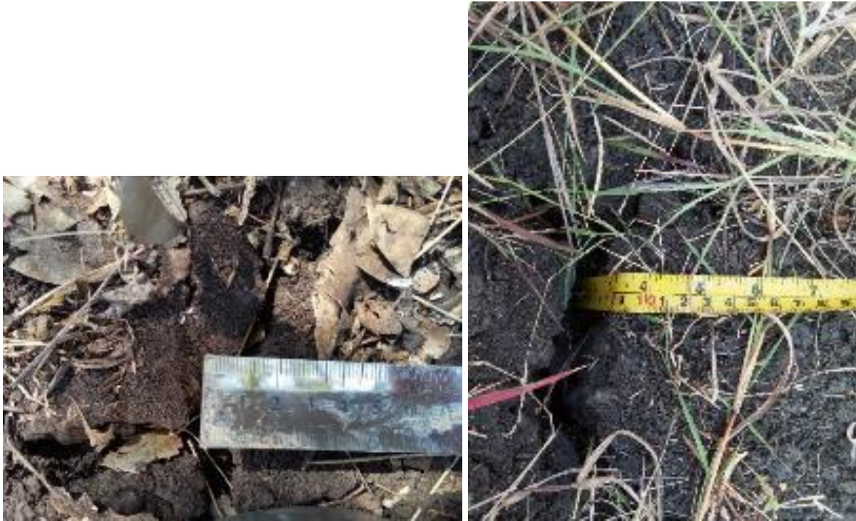
Figure 4.9. Example of desiccation cracks in vertisols of the study area.
