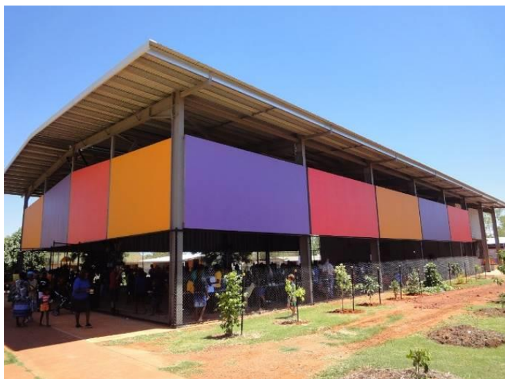
Figure 3.70: Newly built Gymnasium, Lajamanu School
