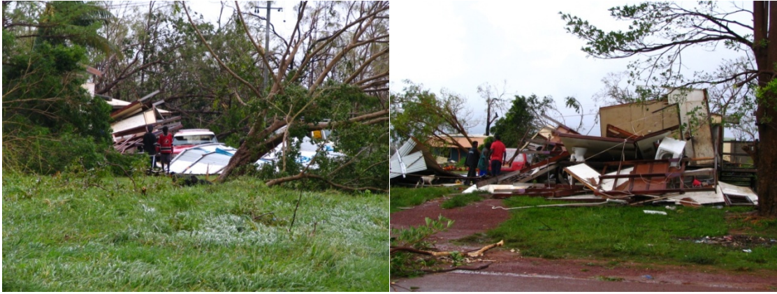
Figure 10.5: Some of the homes that were destroyed in Cyclone Monica. Photo: courtesy of Maningrida Emergency Response Group.
