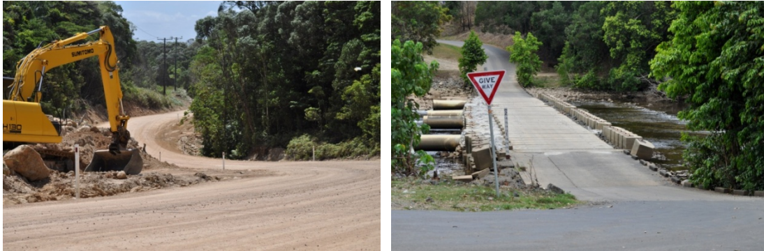
Figure 10.7a: Roadwork between Cooktown and Wujal Wujal to reduce flooding across roadways during the wet season. 10.7b: The temporary causeway across the Bloomfield River linking Wujal Wujal to southern communities and outstations. Photos: Jeanie Govan.
