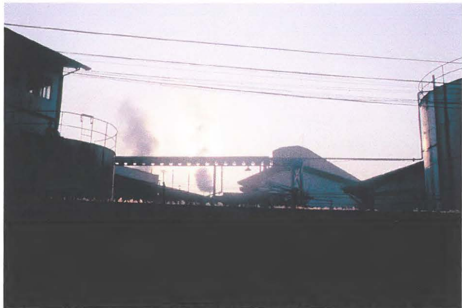
Plate 4.1: A Factory and the Wall (embedded with broken glass) (photo:RWJ)
