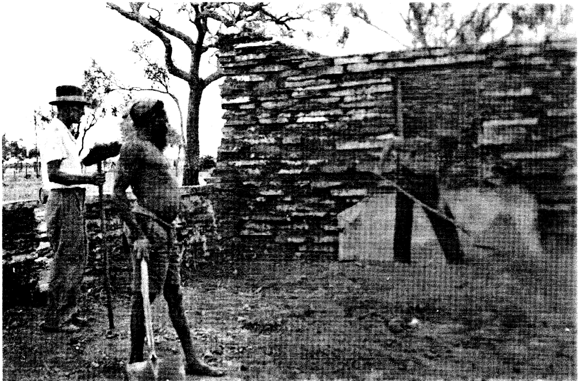
Fig. 2.6 Men employed in building projects, Warburton Ranges Mission 1949
