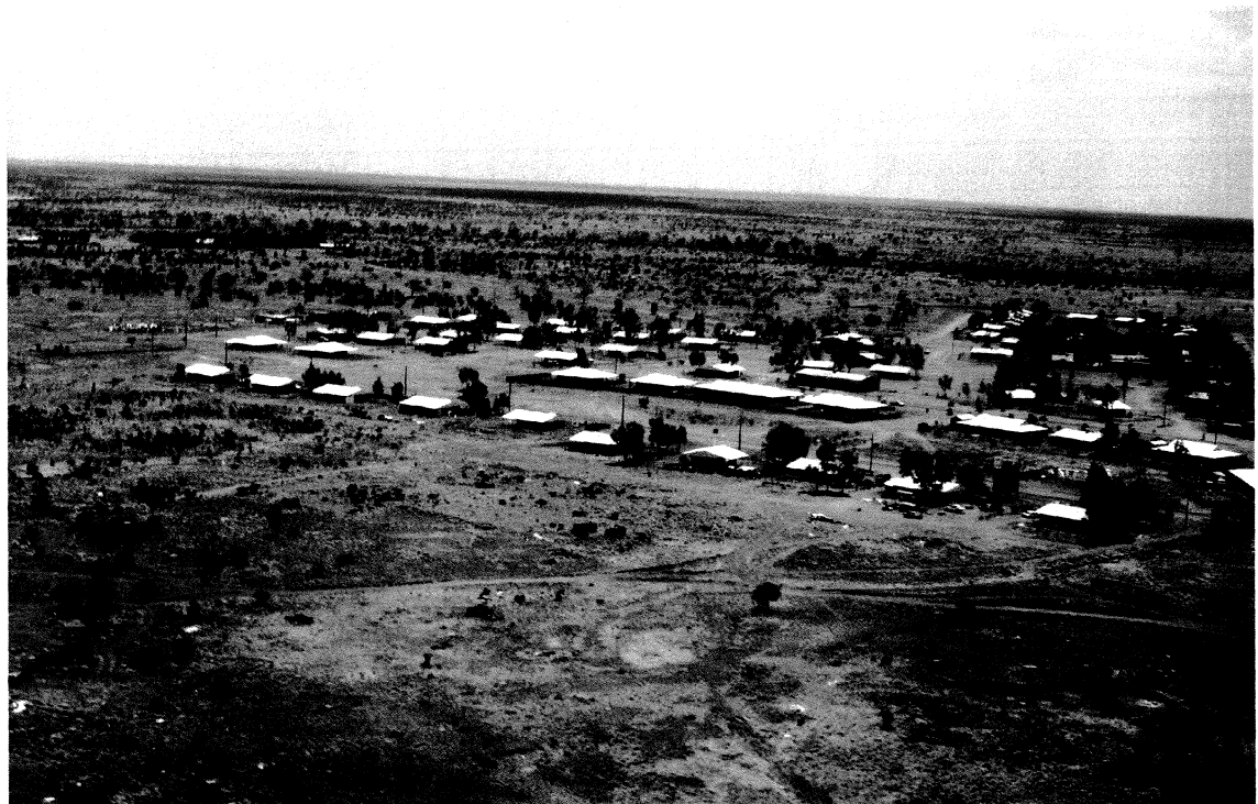
Fig. 1.3 Aerial photo of Warburton 2004
