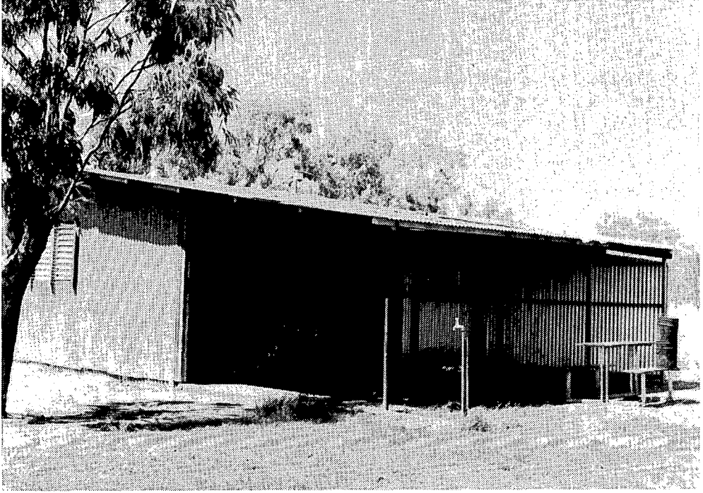
Plate 5: Typical one room camp house. The verandah has been extended to provide more shelter and living space
